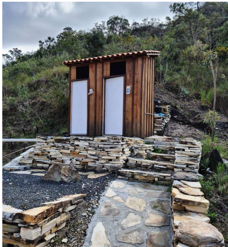
Figure 3 - Toilets with septic tanks in the Complexo do Paraíso Achado.
