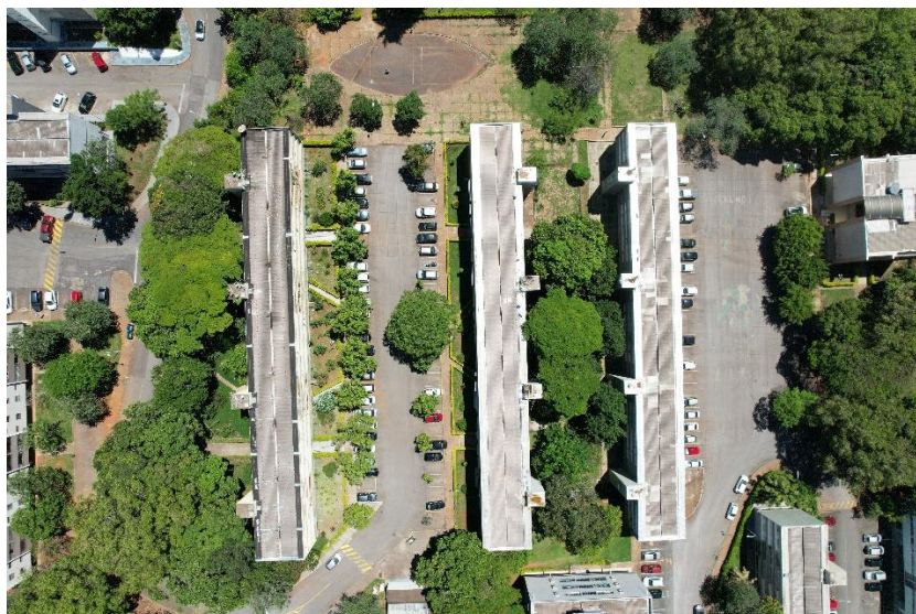
Figure 1 – South Superblock 407 South, South Wing, Brasilia-DF
